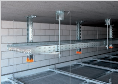
Single-layer ceiling suspension.
