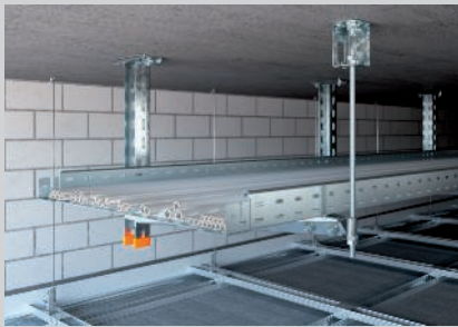
Single-layer ceiling suspension.
