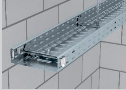
Insertion of the centre suspension in the cable tray.
