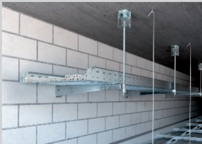
Wall mounting, one and two-layer possible.
