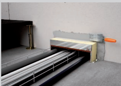
Tidy mortaring in of the box
