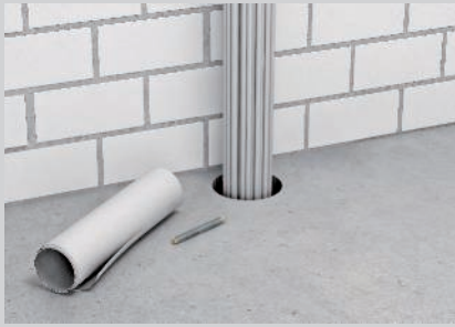
Preparation of the cable insulation.
