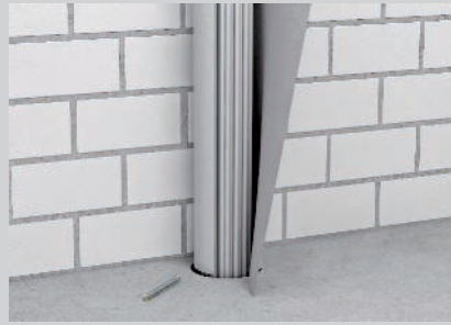
Installation of the fire protection bandage.
