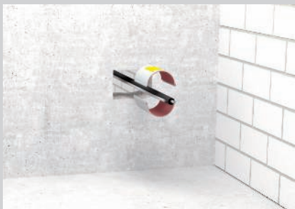
Mounting of the pipe shell by clicking the half shells together around the existing installation.
