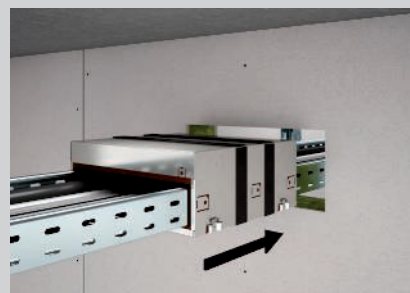
Inserting the box into the wall opening
