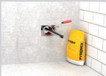
Closing of the opening with PYROMIX® mortar.
