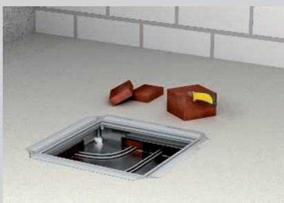
Cut thin strips for the duct compartments.
