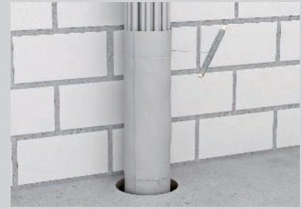
Fixing of the bandage using winding wire.
