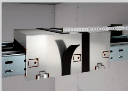
Measuring the wall thickness and attaching graphite strips at the appropriate distance
