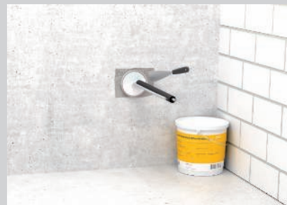
Adjust the foam plugs to installations using a knife and create smoke gas-tight sealing of the sealings using the ASX coating compound.
