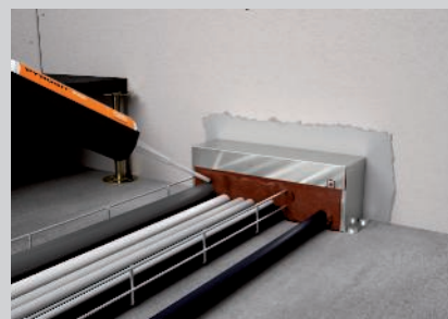
Closing the gaps completely with PYROSIT® NG fire protection foam
