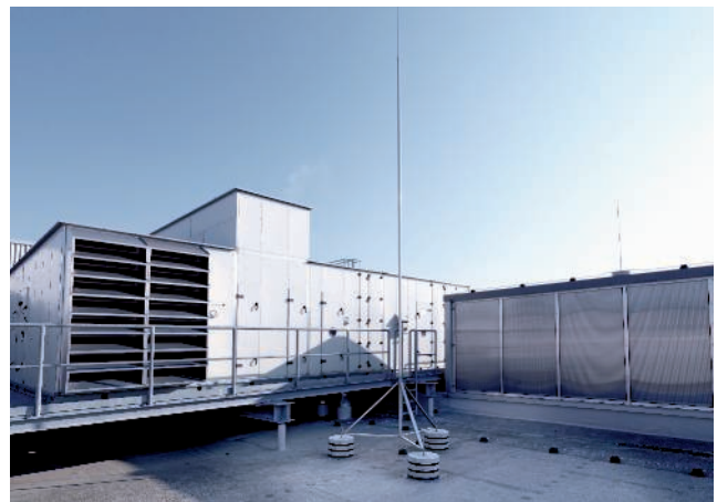
Insulated lightning protection with isFang
