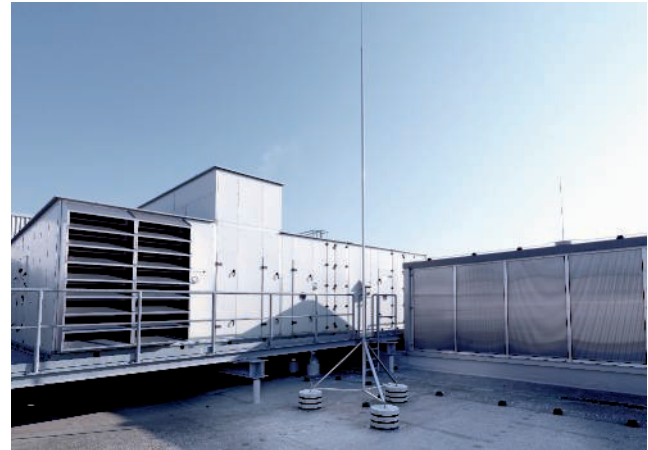
Aluminium air-termination mast
