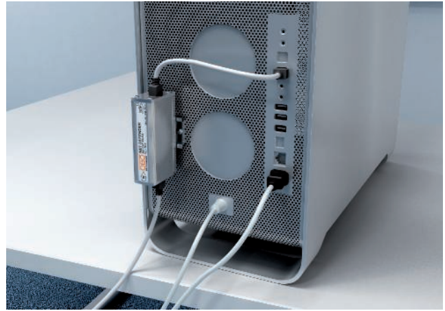
Suggested protection for terminal device. To keep the protection level low, the surge protection device uses the protective conductor of the PC case as the PE connection.
